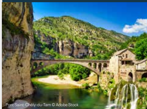
Pont Saint-Chély-du-Tarn © Adobe Stock
